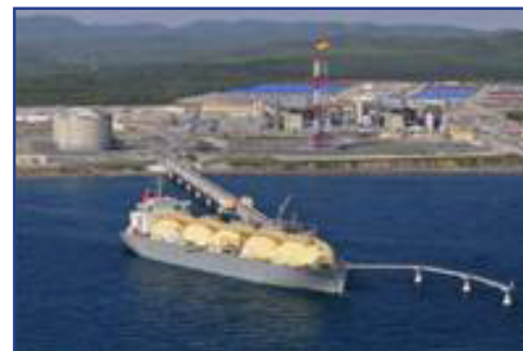
Liquefied natural gas (LNG) plant
